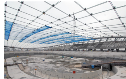
Cable net roof London Velodrome
