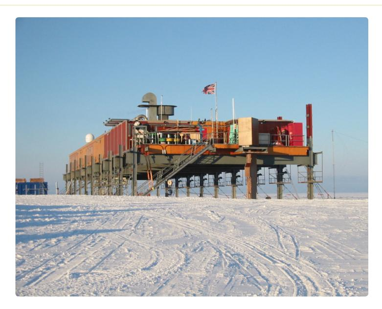
The present Halley V Research Station is a series of science and accommodation platforms raised above the ice surface on jackable legs. There are also two moveable structures on giant skis. The station is the most successful so far in terms of its longevity, use of technology and living experience.
